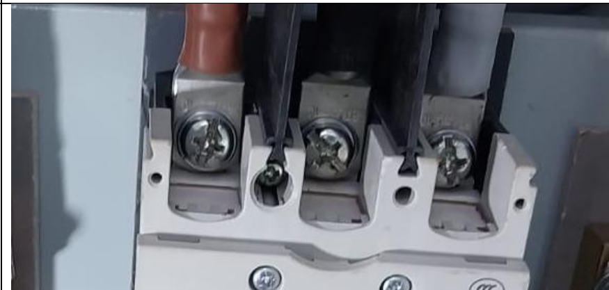
✓ The length of the heat shrink tubes is suitable and should not cover the contact surface of the cable lugs
