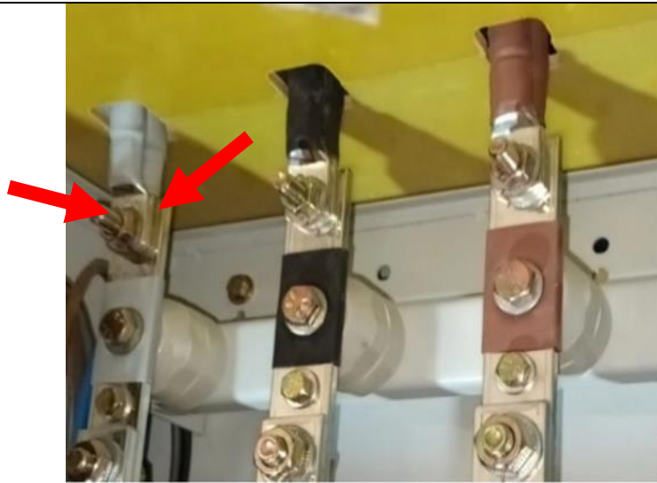
Example 23 : ✖ Incorrect way to connect two cables
