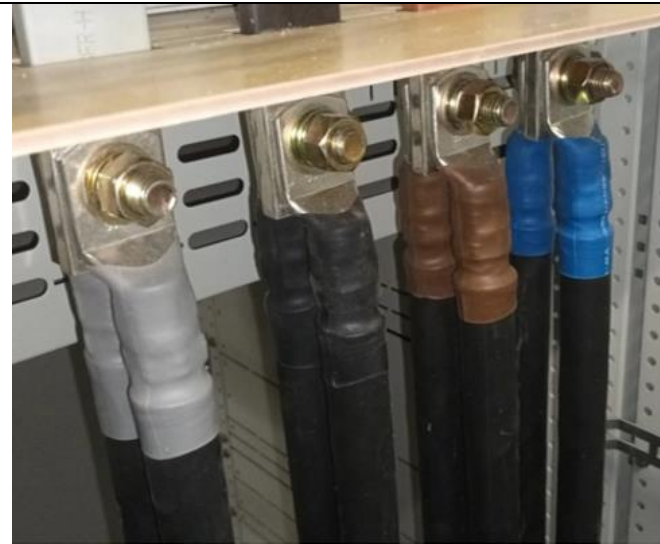
✓ Correct way to connect two cables
